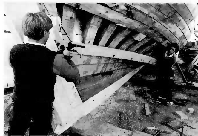
APPRENTICES OF THE MAINE MARITIME MUSEUM'S APPRENTICE SHOP PROGRAM HANG PLANKING ON THE "PINKY" SCHOONER UNDER CONSTRUCTION AT THE MUSEUM'S PERCY & SMALL SHIPYARD IN BATH.
